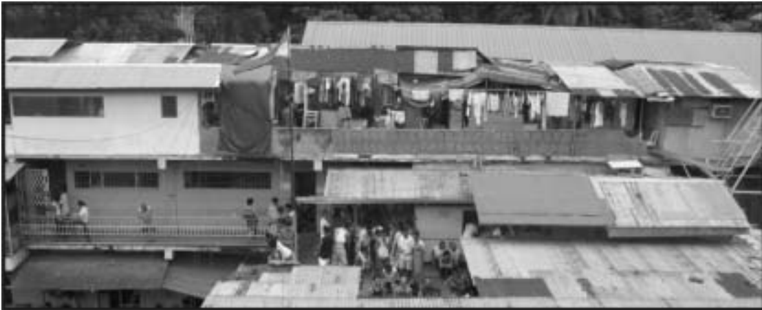
BJMP personnel's offices and living quarters are located on the topmost floor.
