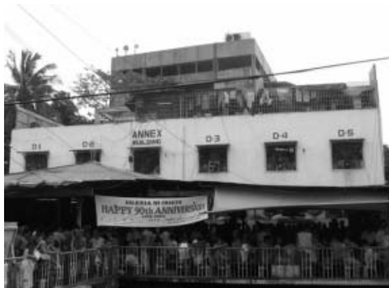
The Annex building is home to members of Querna and the Chinese community (extension, rooftop).
